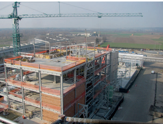
Reverdia facility under construction.
